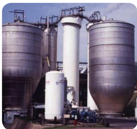
Fig. 5 a) Pulp towers made of 2205
