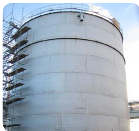
b) white liquor tank made of SAF 2304
