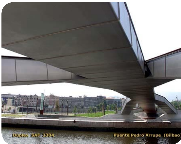
Fig. 8 Bridges for pedestrians and cyclists in Bilbao (left) and Stockholm (right) made of SAF 2304 and 2205 respectively.
