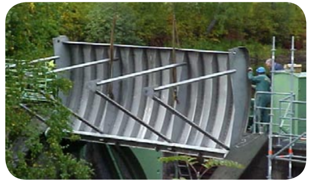
Fig. 10 Footbridge along a Norwegian mountain track (left) and a floodgate in Sweden (right), both made of LDX 2101.
