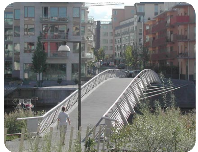
Fig. 8 Bridges for pedestrians and cyclists in Bilbao (left) and Stockholm (right) made of SAF 2304 and 2205 respectively.
